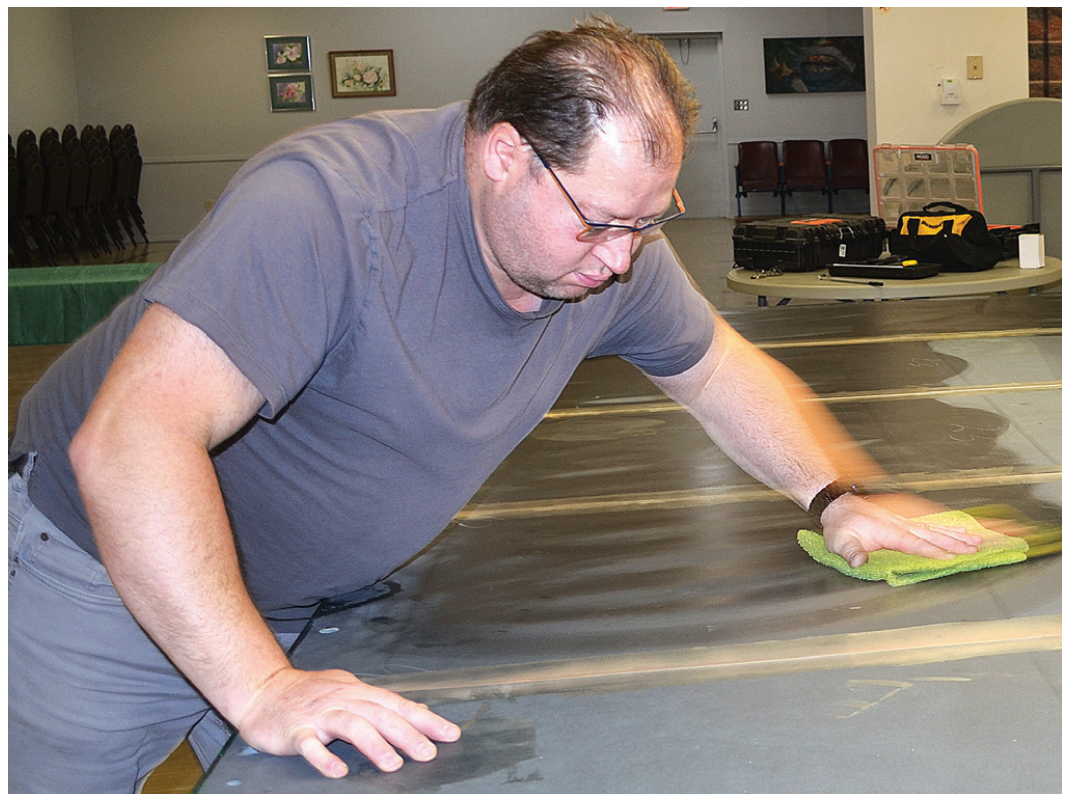
Snooker table repairman Mike Wasoyliw cleans and levels off the shale which makes the 2,000 lb. table so heavy. PATRICIA HARCOURT PHOTOS
