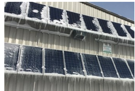
Photo: Wall mounted solar panels outside an arena in Iqaluit, NU, http://www.cbc.ca/news/canada/north/iqaluit-arena-has-new-solar-panels-1.3499877
